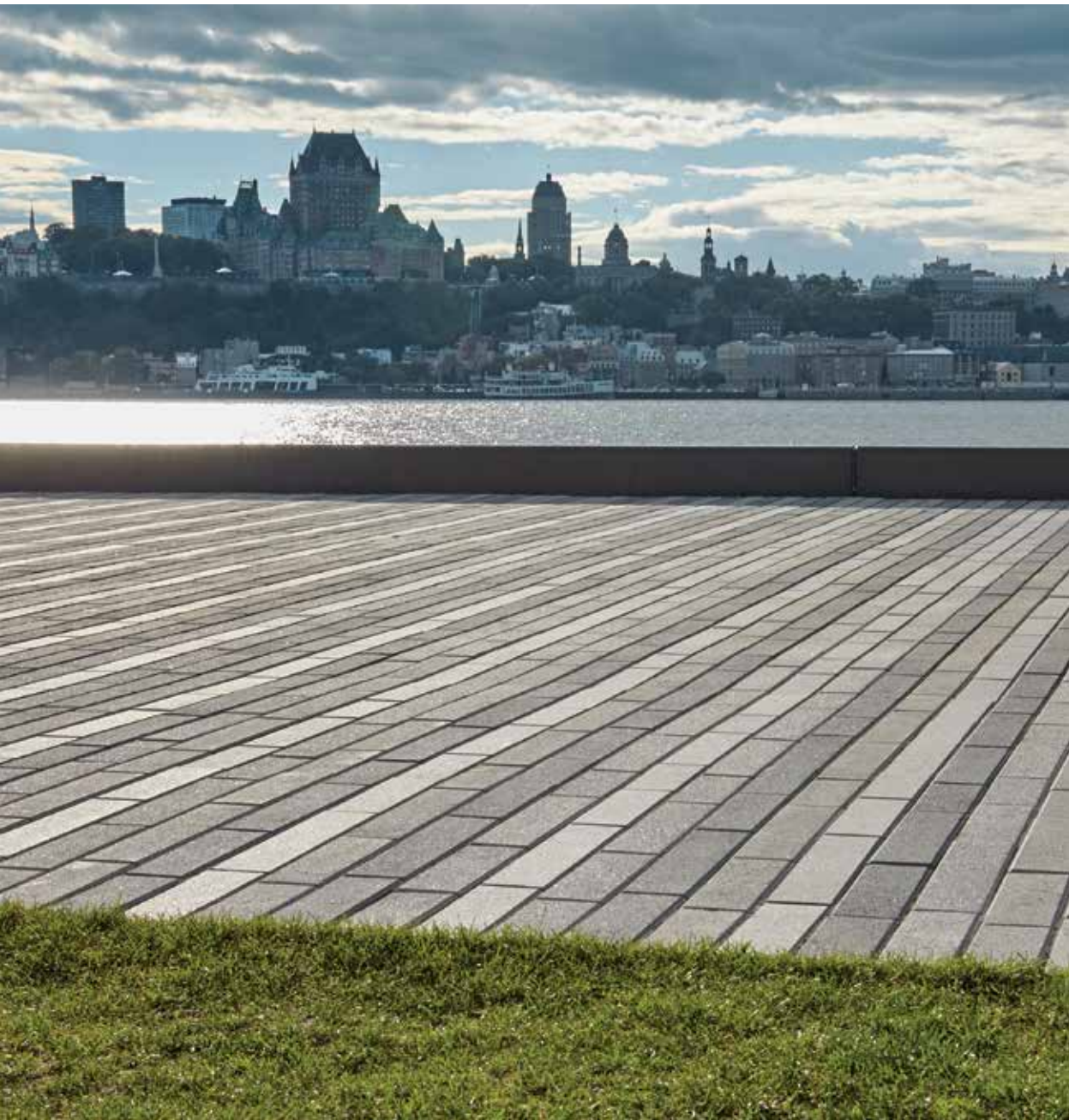
Rehabilitation of the Paquet Warf, Lévis BOULEVARD TLI 150 CRESCENDO 125
