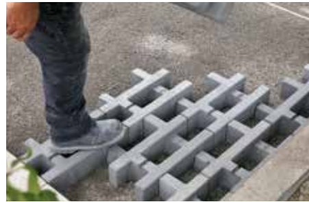
Boulevard Verde pavers are laid in strips on a conventional densified granular foundation.
