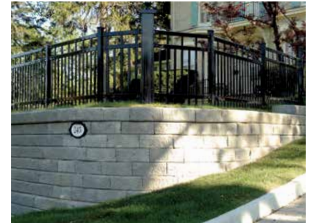
Grande walls allow for curved designs
