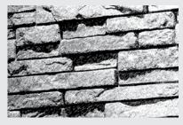
Once the installation is complete, clean the wall thoroughly with a stiff brush in order to remove any excess mortar. Remove any residue in the "inner joint in. with a trowel, a thin jointing tool or any other similar tool. Leave wall to dry for approximately 24 hours or until completely dry. Wash with any stone or masonry cleaner recommended by Permacon. Repeat this last step as needed.
