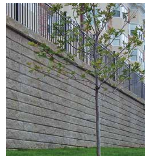
Fence incorporated directly above wall
